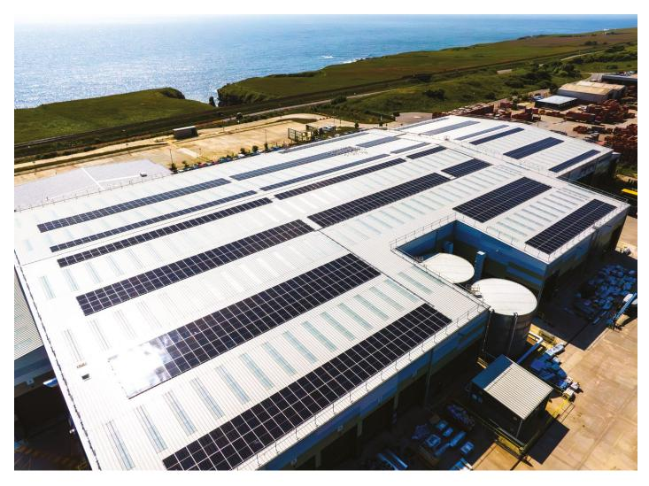
Roof with non-fragile rooflights and PV panels in perfect harmony without the need for rooflight covers.
