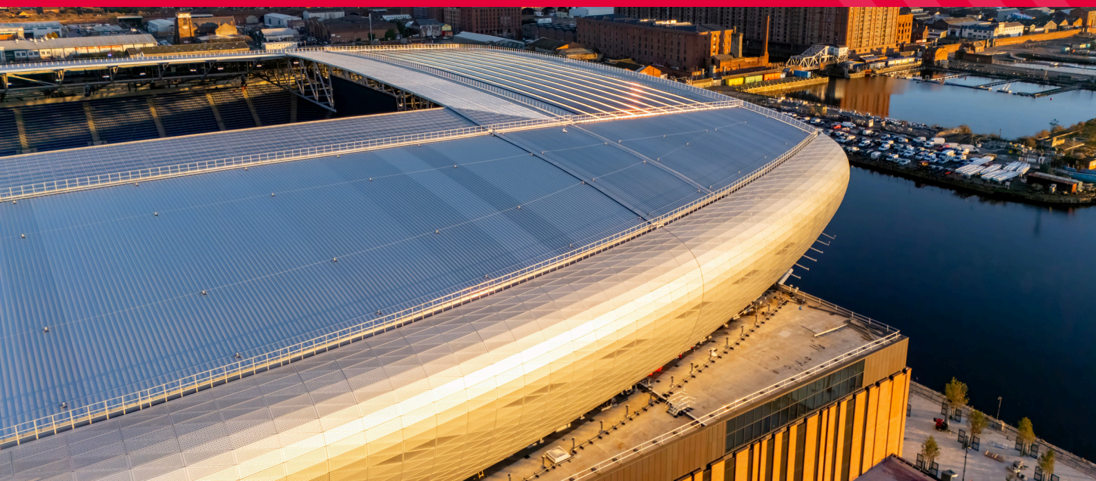
Sheeting & Cladding, Hill Dickinson Stadium
