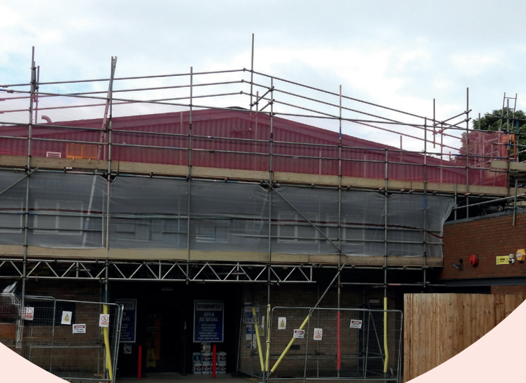
Figure 1: Store frontage scaffolding to allow public access to and from the store
