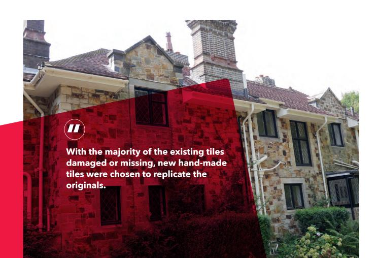
This 18th century Grade II listed landmark needed a full restoration, so Richardson Roofing were contracted to strip off and renew the Welsh slates and the sheet copper weathering. Copper to the cupola and the flat roofs were retained, with intricate repairs made at the request of the architect.
