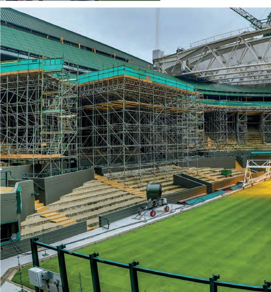
Prater's scope of works was to deliver an extensive roofing package for the iconic No.1 Court at Wimbledon, making it an all-weather tennis arena. The project, which was divided into three phases to enable the venue to carry on functioning, also sought to increase overall seating capacity to 12,4000 by adding two new seating tiers. This required significant supporting structural steel frames.
