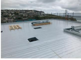
Pools on the rooftop terrace of this concrete residential block had been leaking into the basement car park, so Makers Construction had to drain the 148,000 litres of water, plus accumulated silt before installing robust waterproofing.
