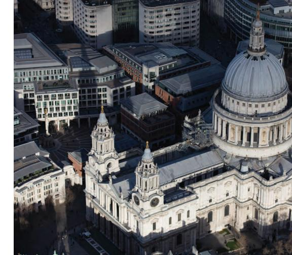
Sussex Asphalte renewed the existing asphalt to the North Courtyard, replacing the 500sqm of existing asphalt, due to water ingress affecting the Cathedral's workshops and storage facilities. By recycling the 100-year-old asphalt, stripped from a previous project on the Stone Gallery, the team saved St Paul's Cathedral, over £11,000 in costs.
